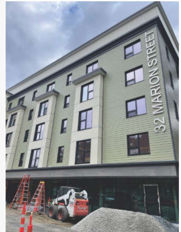
Construction in progress at 32 Marion Street, photo courtesy of Delphi Construction, Inc.
