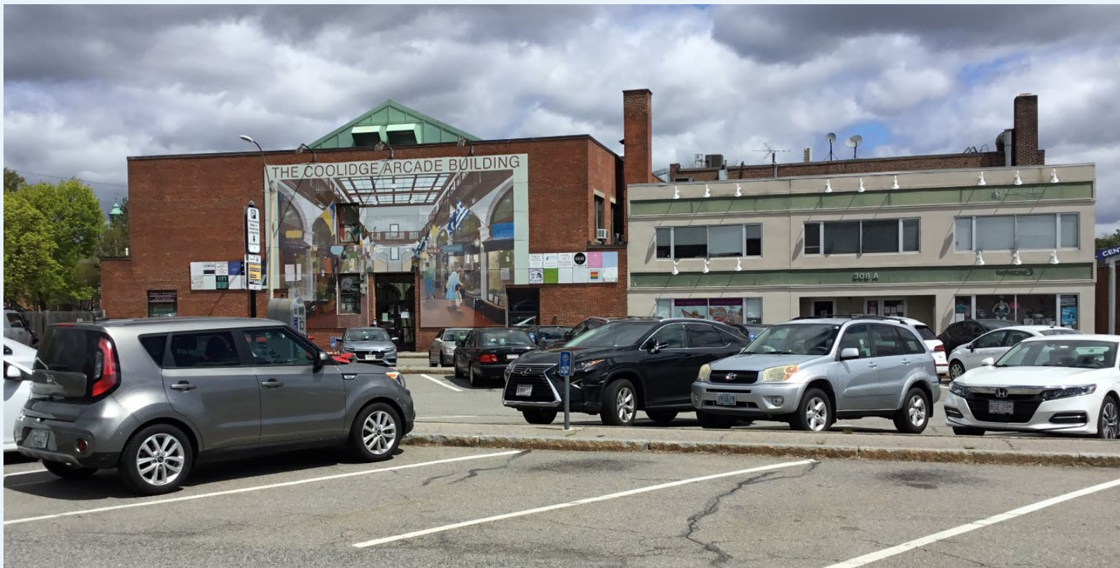
Existing Condition: Centre Street Municipal Parking Lot, Brookline, MA (April 2021)
