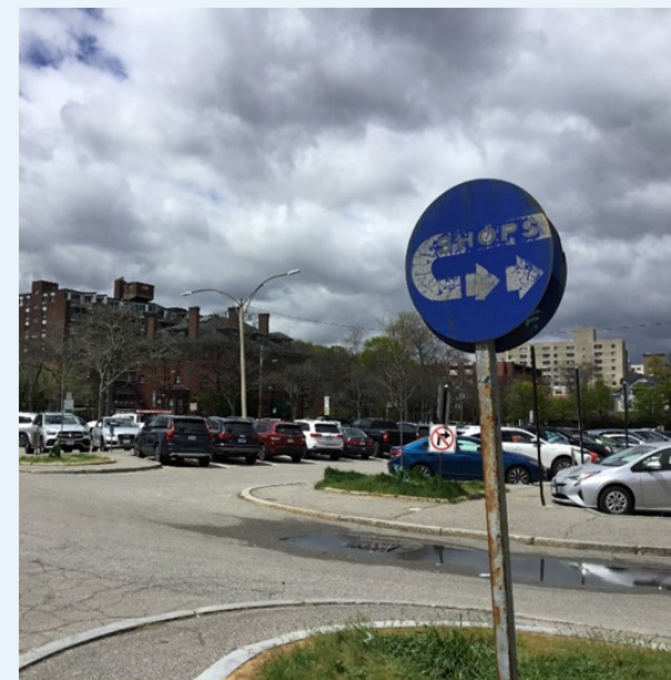
Existing Condition: Centre Street Municipal Parking Lot, Brookline, MA (April 2021)
